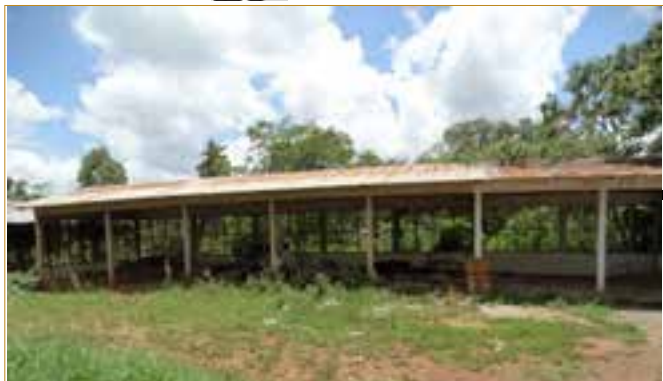
Previously a cow shed for storing fodder
