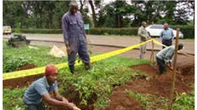
The Installation of Local Area Network (LAN)
