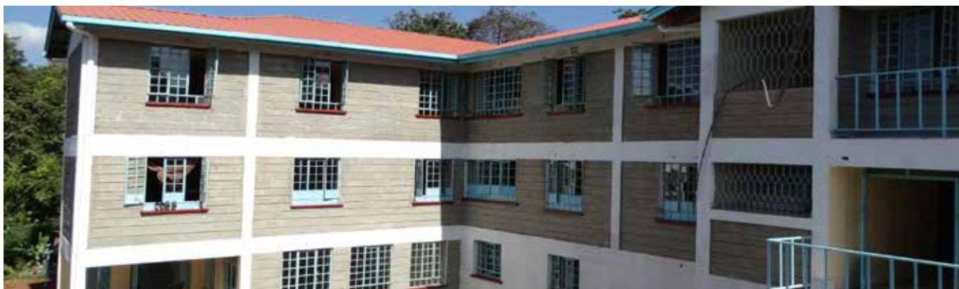
Mt. Kilimanjaro Hostel, one of the newly constructed female hostels.
