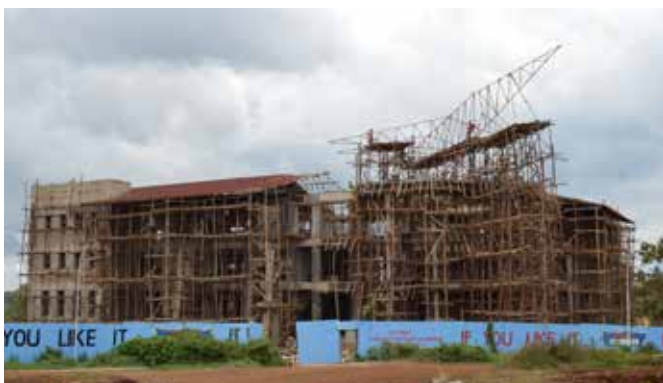
Modern Library Under Construction
