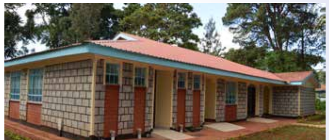
The newly completed University Guest House
