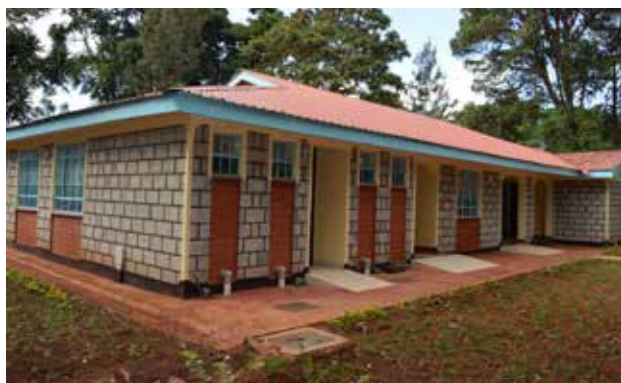
The newly completed University Guest house.
