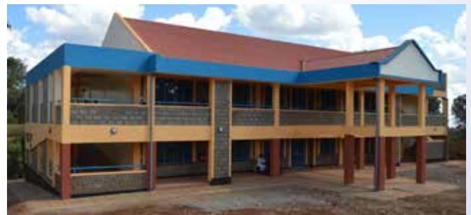
The newly completed Office Block
