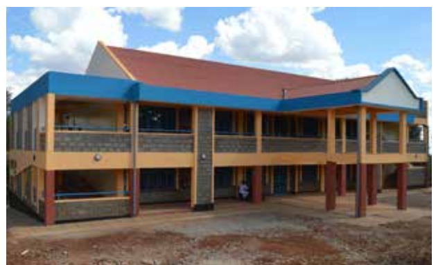
The newly completed Office Block.
